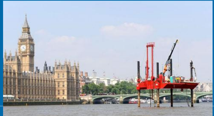
Drilling rig carrying out exploratory work on the Thames
